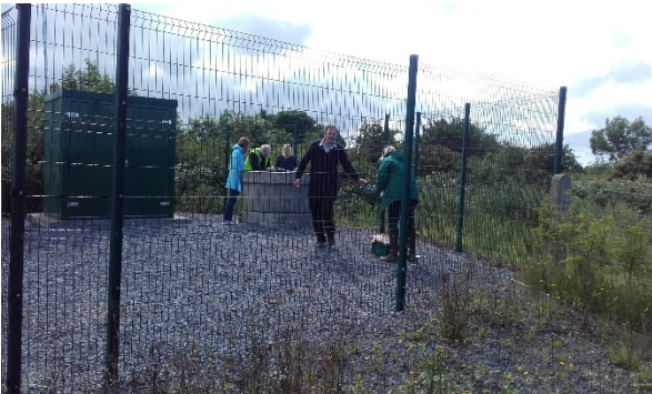
Photo 3. BH1 fenced compound and pump chamber
