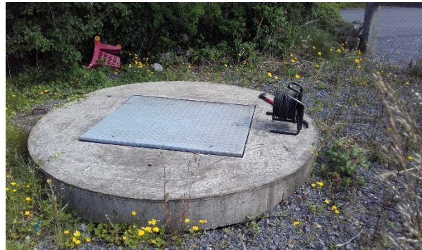
Photo 4. BH2 chamber and adjacent road
