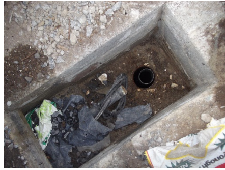
Photo 2. BH2 below ground level in chamber.
