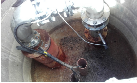
Photo 1. BH1 pump and rising main in pump chamber
