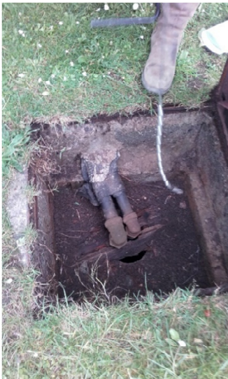
Photo 5. Open borehole, below ground level in Kiltiernan national school grounds.
