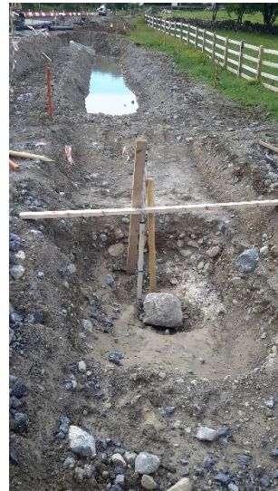
Photo 6. Infiltration trenches along N18 interchange, north east of Kiltiernan N.S.
